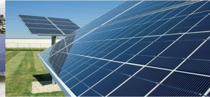
**FOAM OR SALVAGE COVER** – You cannot block the sunlight on the PV array with foam or a salvage cover. Foam will slide off the PV array, and although a salvage cover significantly reduces sunlight to the array, electricity can still be generated through it.
