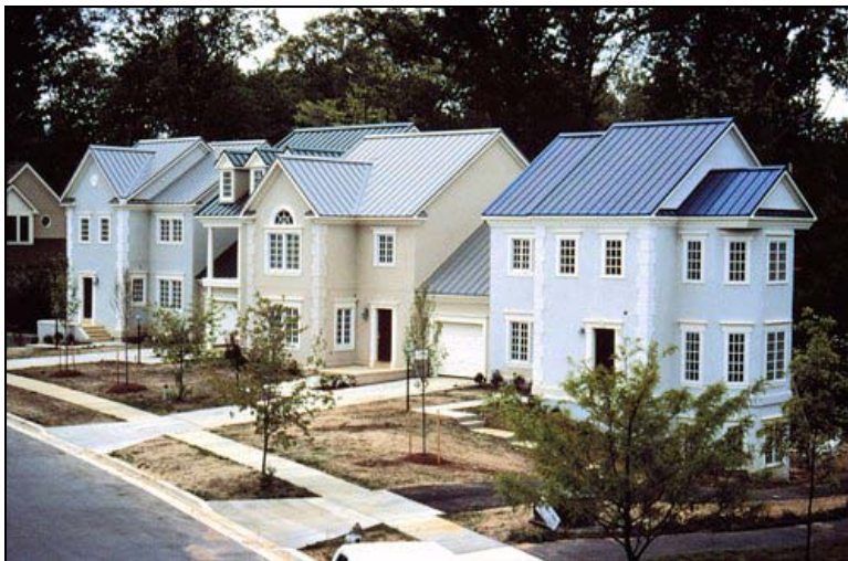
Figure 5-4: Townhouse with PV Systems in Maryland (Photo courtesy of NREL Photographic Information Exchange)
