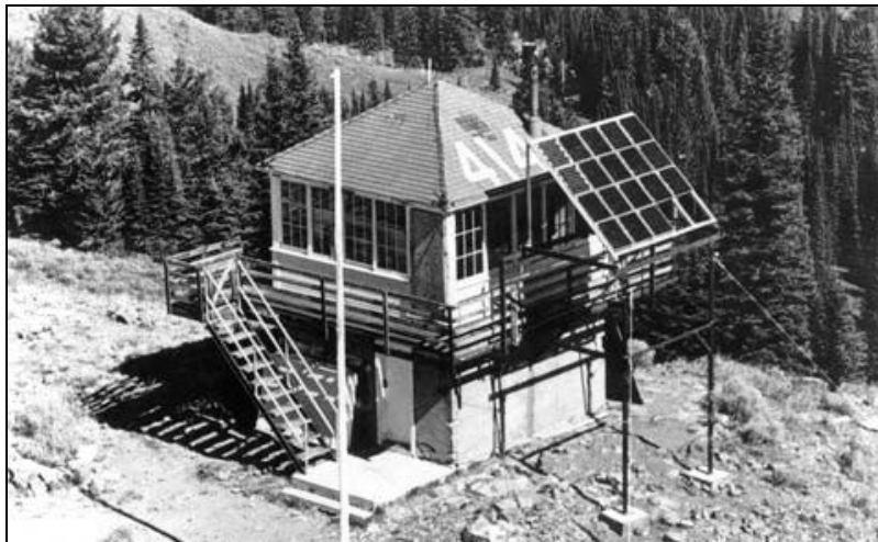
Figure 2-8: Example of PV System at a Remote Fire Lookout Tower in Idaho (Photo courtesy of NREL Photographic Information Exchange)
