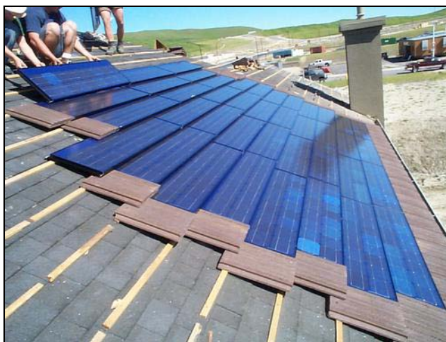
Figure 3-5: Example of PV Roof Panels Shaped Like Conventional Roofing Shingles (Photo courtesy of NREL Photographic Information Exchange)
