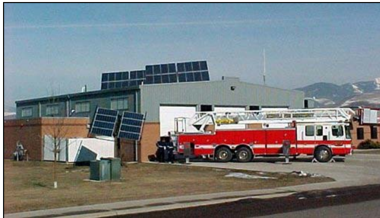
Figure 2-7: Example of Fire Station with a Photovoltaic Solar Power System in Missoula, MT (Photo courtesy of NREL Photographic Information Exchange)
