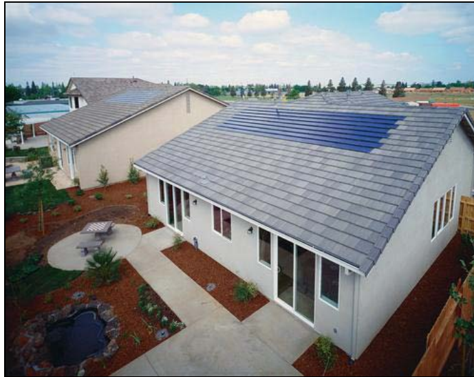
Figure 5-2: Residential Occupancy with a PV System Integral to the Roof Assembly (Photo courtesy of NREL Photographic Information Exchange)
